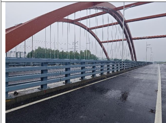
淠河总干渠大桥防撞栏
